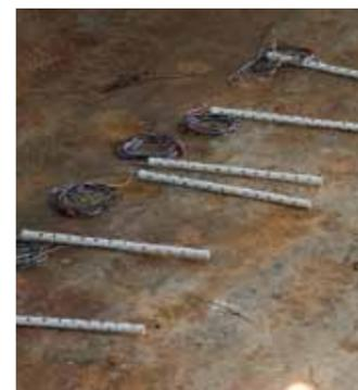
Assembled ICCP anodes (in perforated PVC protective sleeves) lie on a barge awaiting installation, above. At right, Lance Thomas of Anode Solutions crimps cable connections for the *USS Midway*. The final result, far right, is 30 anodes protecting the hull of the aircraft carrier against exterior corrosion. Not huge in size, but mighty in their power.
